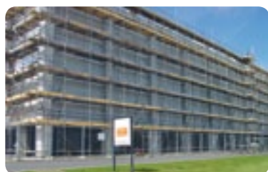
Figure 5: Scaffolding on a multi-storey building.
